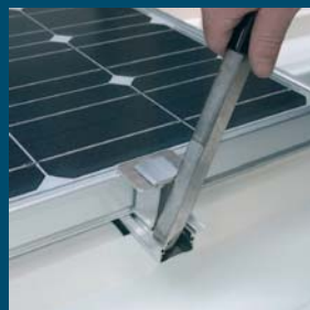
Fixing the SCG 3.0 module retainers with bending gage
