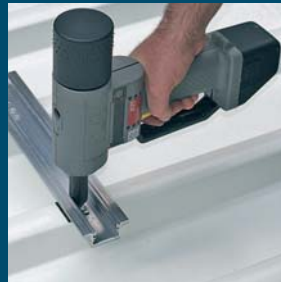
Riveting the carrier profile with seal to high bead
