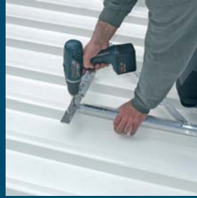
Drilling with drill jig
